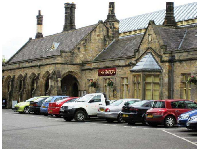
The Station and upper car park
